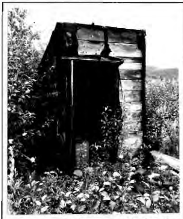
Figure 157. The Generator Shed, 1993. The view is looking north.
